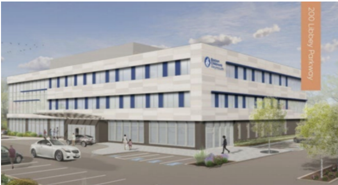
200 Libbey Industrial Way, Weymouth MA 69,000 SF, Off Campus MOB leased by Boston Childrens Owned/Developed by Foxrock Properties LLC Started 1Q2022
